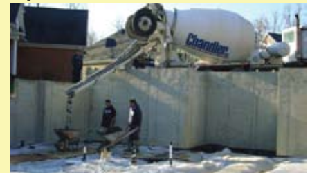
Pouring a basement footing for Jose Juarez and Best Builders.
