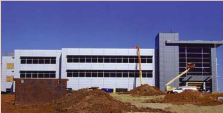
Honda Jet at Greensboro Airport, JMW Concrete
