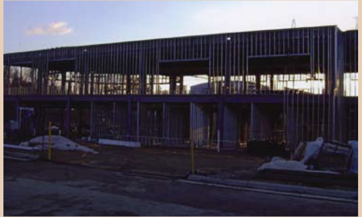
GTCC Classroom Wendover Campus Bar Construction
