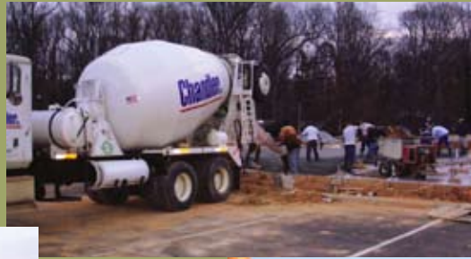
Pouring continues at the Manning Park project
