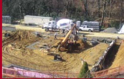
The Medical Center project with Hickory Construction in Boone
