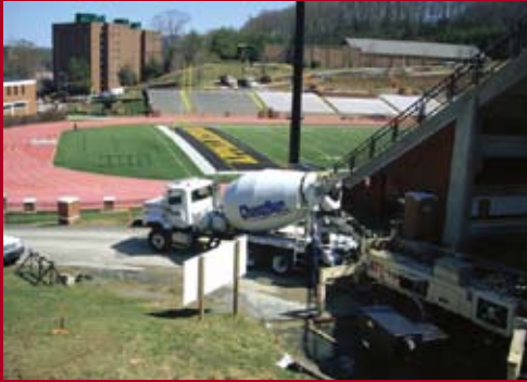
Another load delivered to the Appalachian State football stadium project
